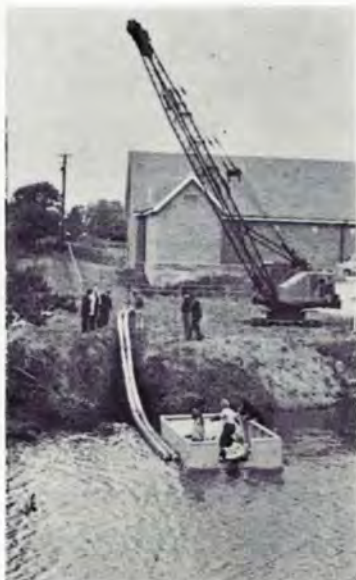
Twin PVC tubes lowered on to the water ready for drawing across.
