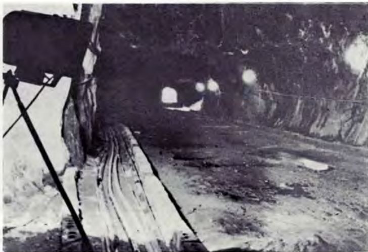
Halogen lamps light up one of the tunnels through the mountain in which our cables are laid in channels on either side. Some 24 hours after this picture was taken thousands of tons of slate roared down the mountain-side blocking off one end of the tunnel.
